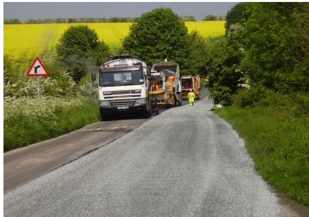
Image One – Chippings being applied
